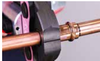
2. Complete the joint with the approved tool. Press once only
