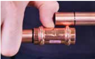
7B. Check the depth mark
