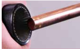
2. Deburr and remove all external sharp edges
